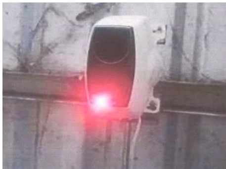
Smoke Beam Detector
